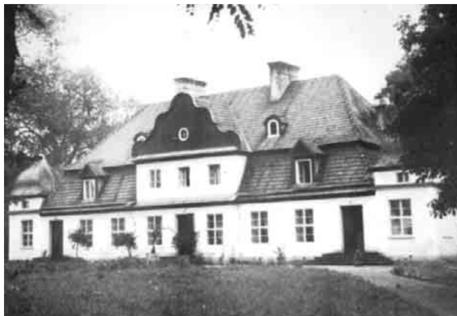
Fig. 5 Brick manor house in Koszuty after renovation (photo: Rydel M., Rydel 1993)
