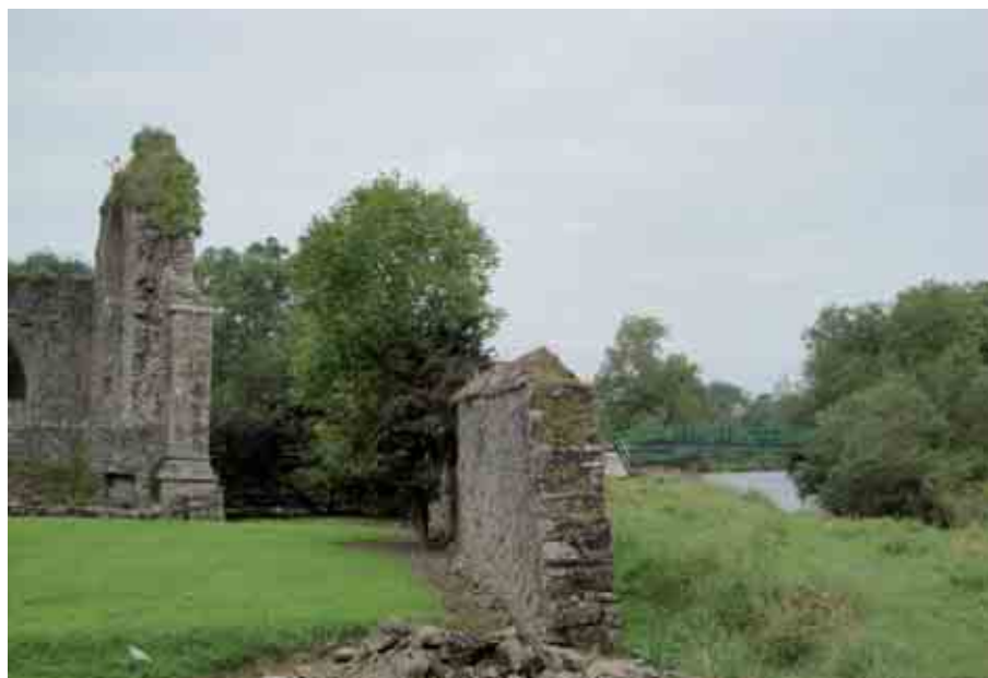
Fig. 5 The breach in the walls facing towards the river
