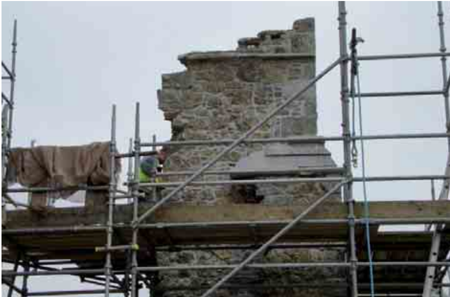
Fig. 10 Restoration of the corner wall of the choir in the church
