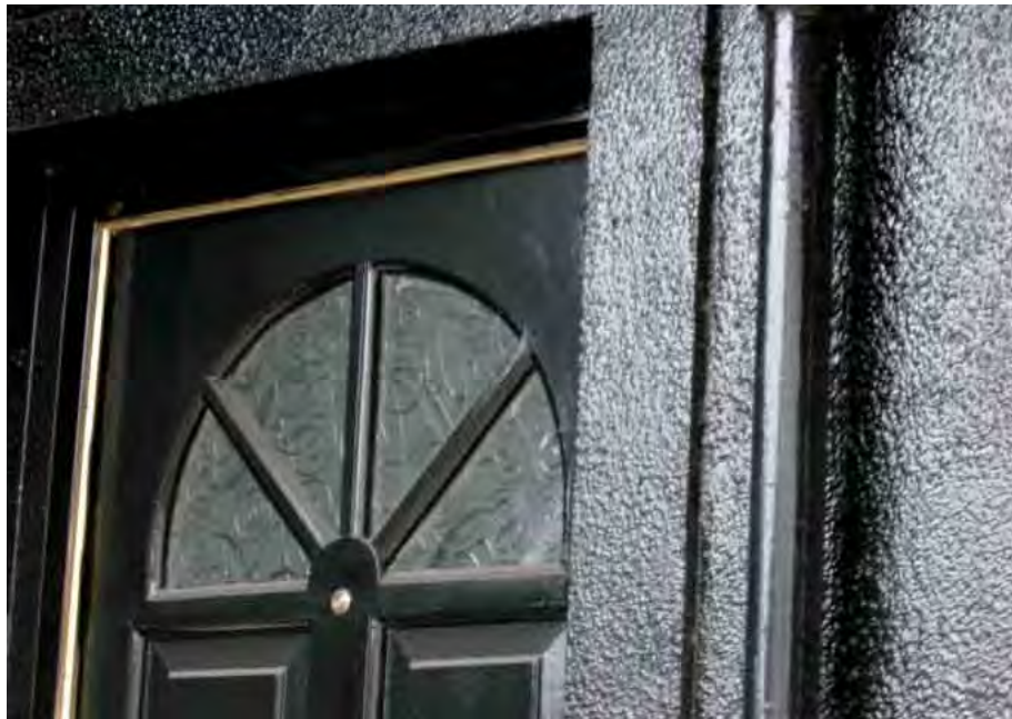
Figg. 7, 8 Widespread superficial finishes of the ground floor and other floors, extraneous to the historical context
