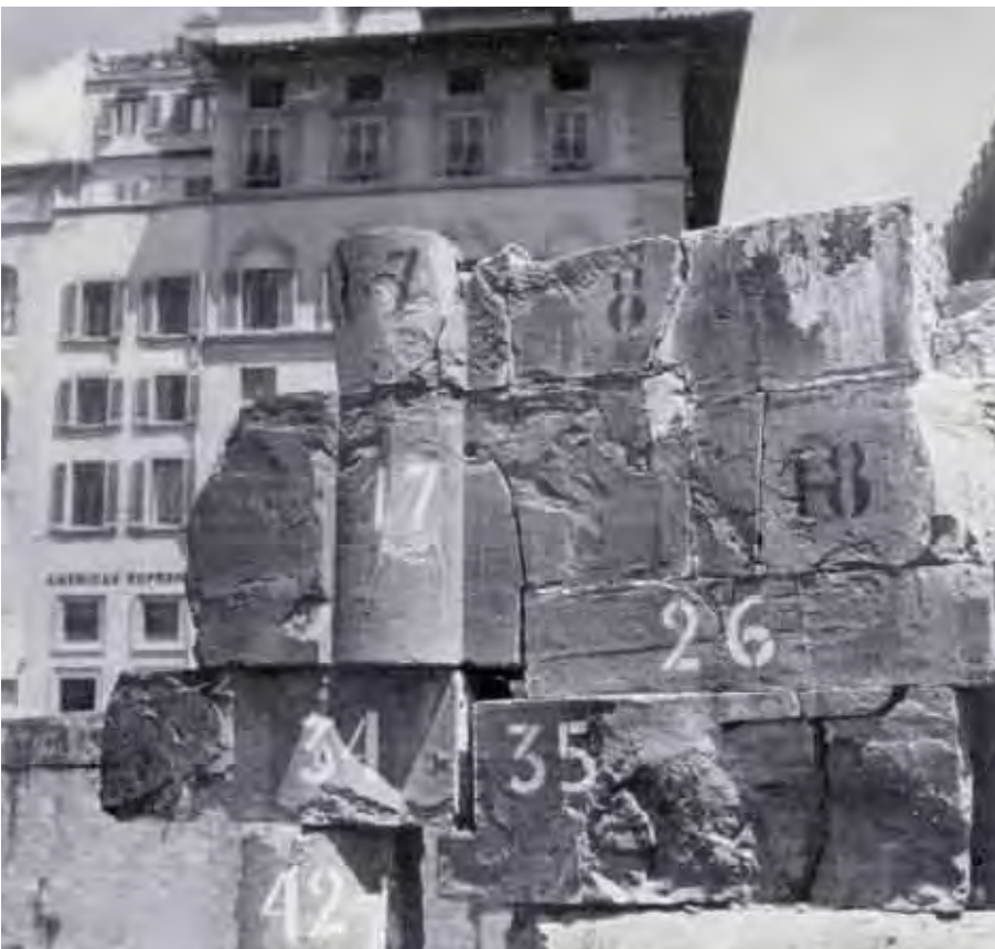
Fig. 5 Ashlar stones of the revetment numbered before dismantling
