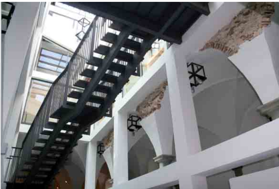
Fig. 24 The new metal staircase and the relicts of the vaults left exposed to view.
