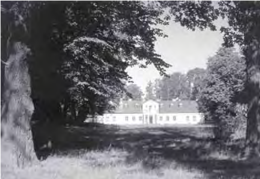
Fig. 1 Landscape setting - manor house in Nagłowice (photo: Markowski S., Markowski 1996)
