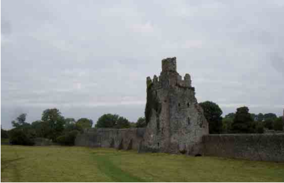
Fig. 4 Kells, Ireland, Augustinian Priory, general views of the site
