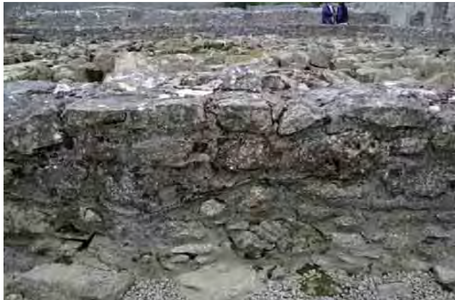
Fig. 7 Sheathing between the reinforcement/ protection layer and the layer of wall beneath
