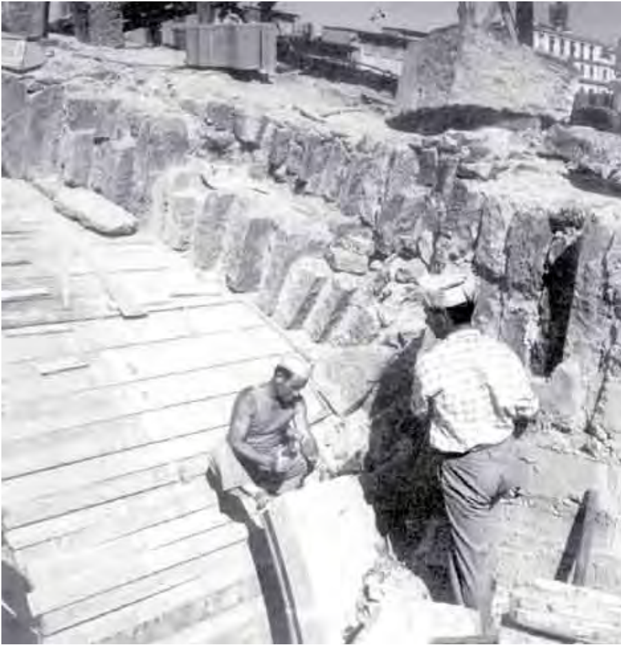
Fig. 12 The springing of an arch during the reconstruction
