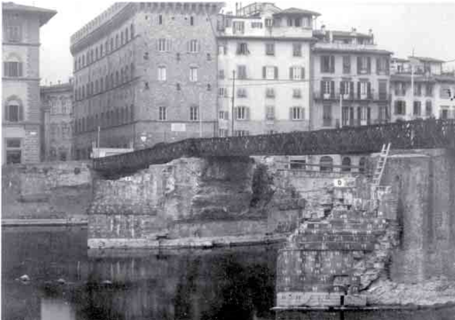
Fig. 4 The remnants of the piers supporting the Bailey Bridge, built for the passage of the Allied forces
