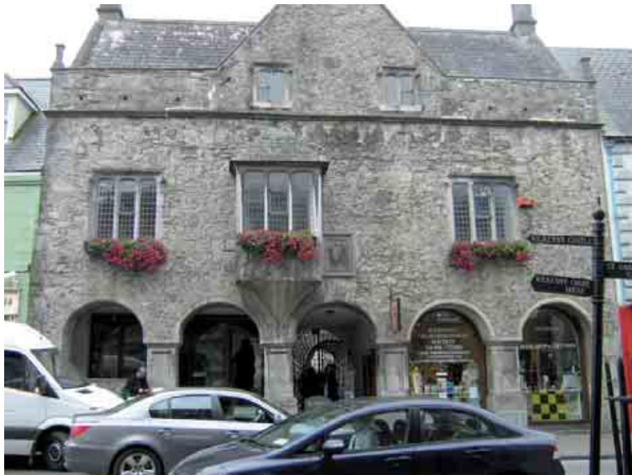
Fig. 5 Rothe House: the façade on High Street
