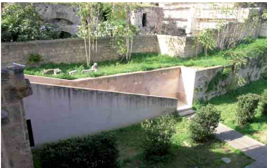
Fig. 11 Palermo, 'Palazzo Belmonte-Riso'. New staircase of access to the palace from the garden
