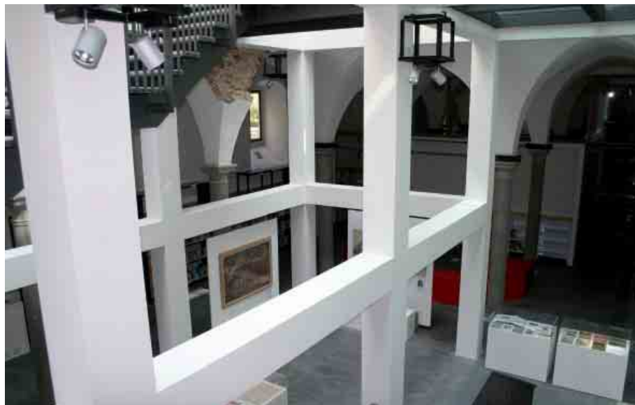
Fig. 22 The new frame on the ground floor.
