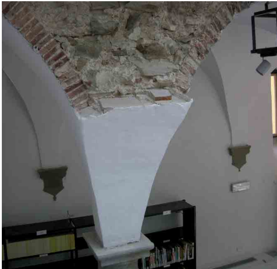
Fig. 25 Details of a vault springing
