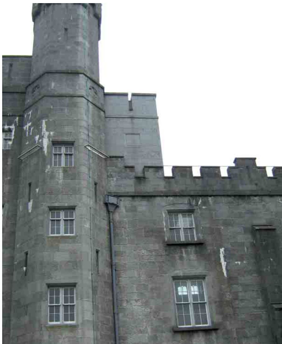
Fig. 12 Kilkenny Castle: the headroom of the lift on the roof
