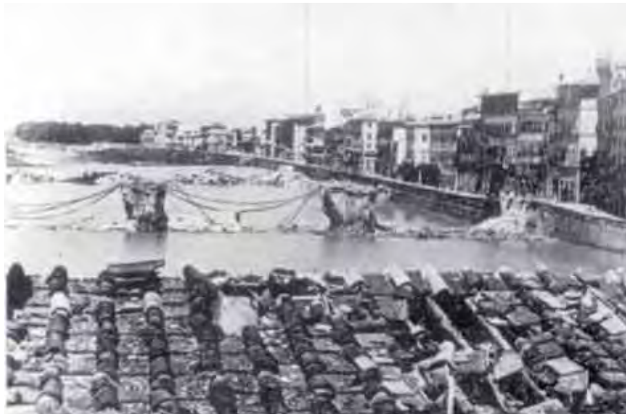
Fig. 2 The Santa Trinita Bridge after the destruction caused by German mines
