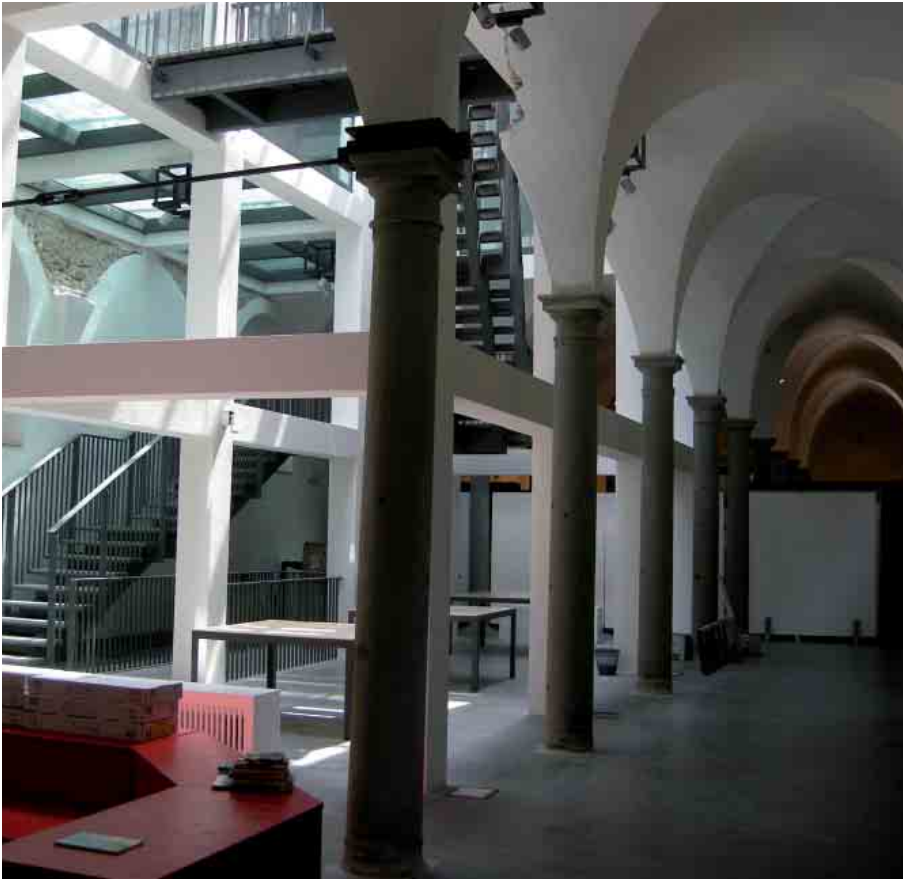
Fig. 23 The new structure, columns and vaults of the remaining aisle
