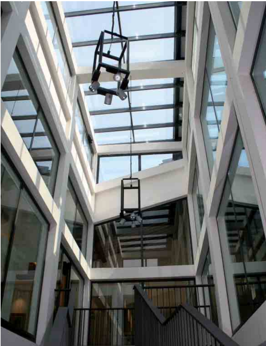
Fig. 20 The reinforced concrete frame with glazing that encloses the upper floors.
