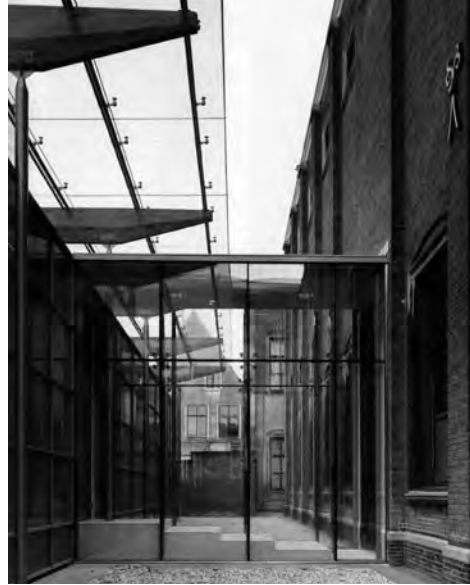
Fig. 9 Teylers Museum, Haarlem, Netherlands, renovation architect Hubert-Jan Henket, 1993-2002.
